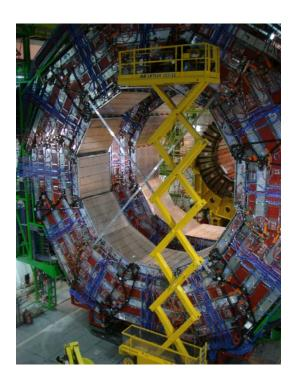
Figure 220: Installation of the MABs on wheel YB+2.
