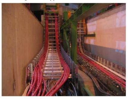
Figure 251: YB+2 and YE+1 cable-chains in UXC55 basement trenches.
