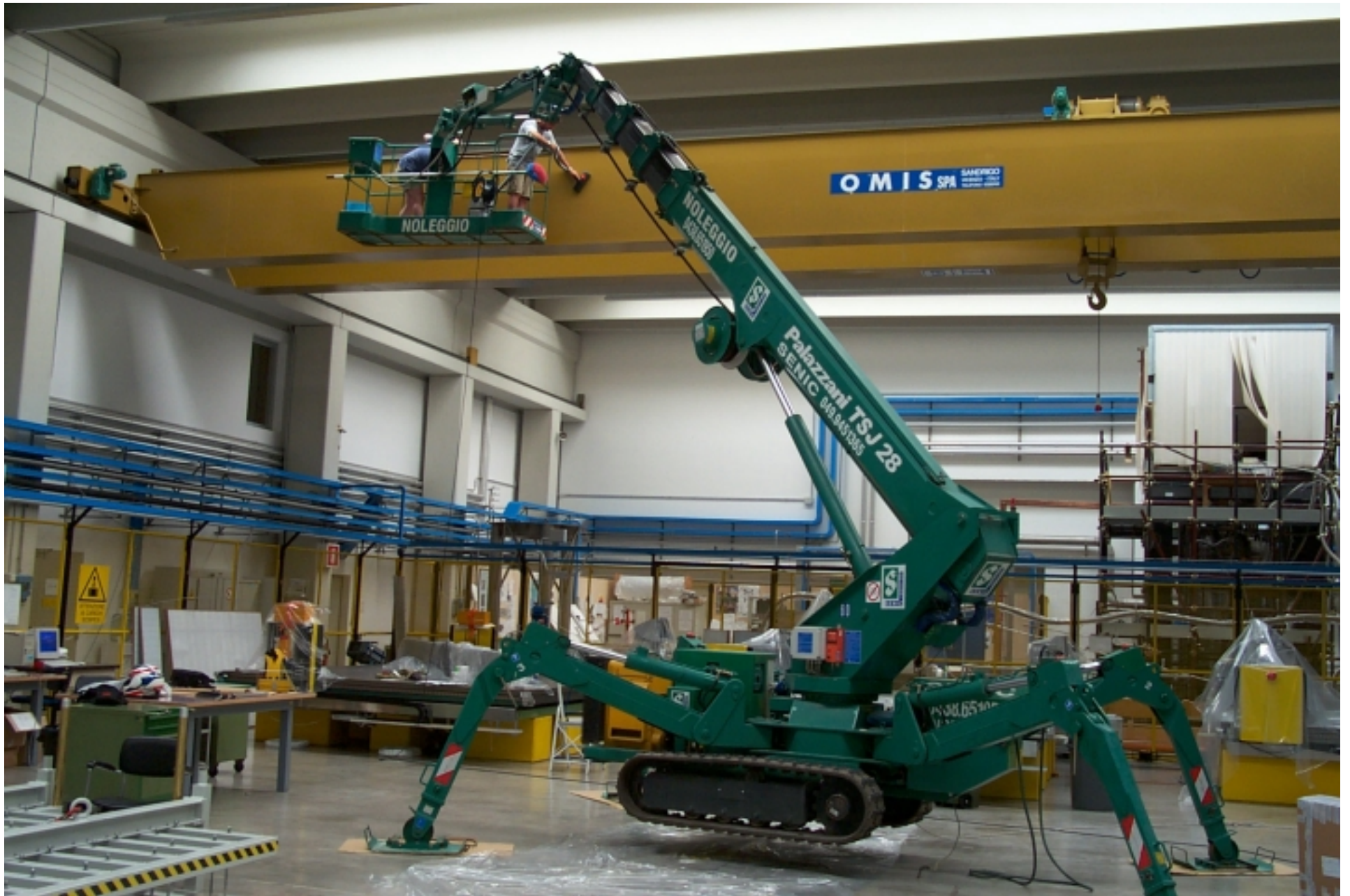
Cleaning of Legnaro hall
