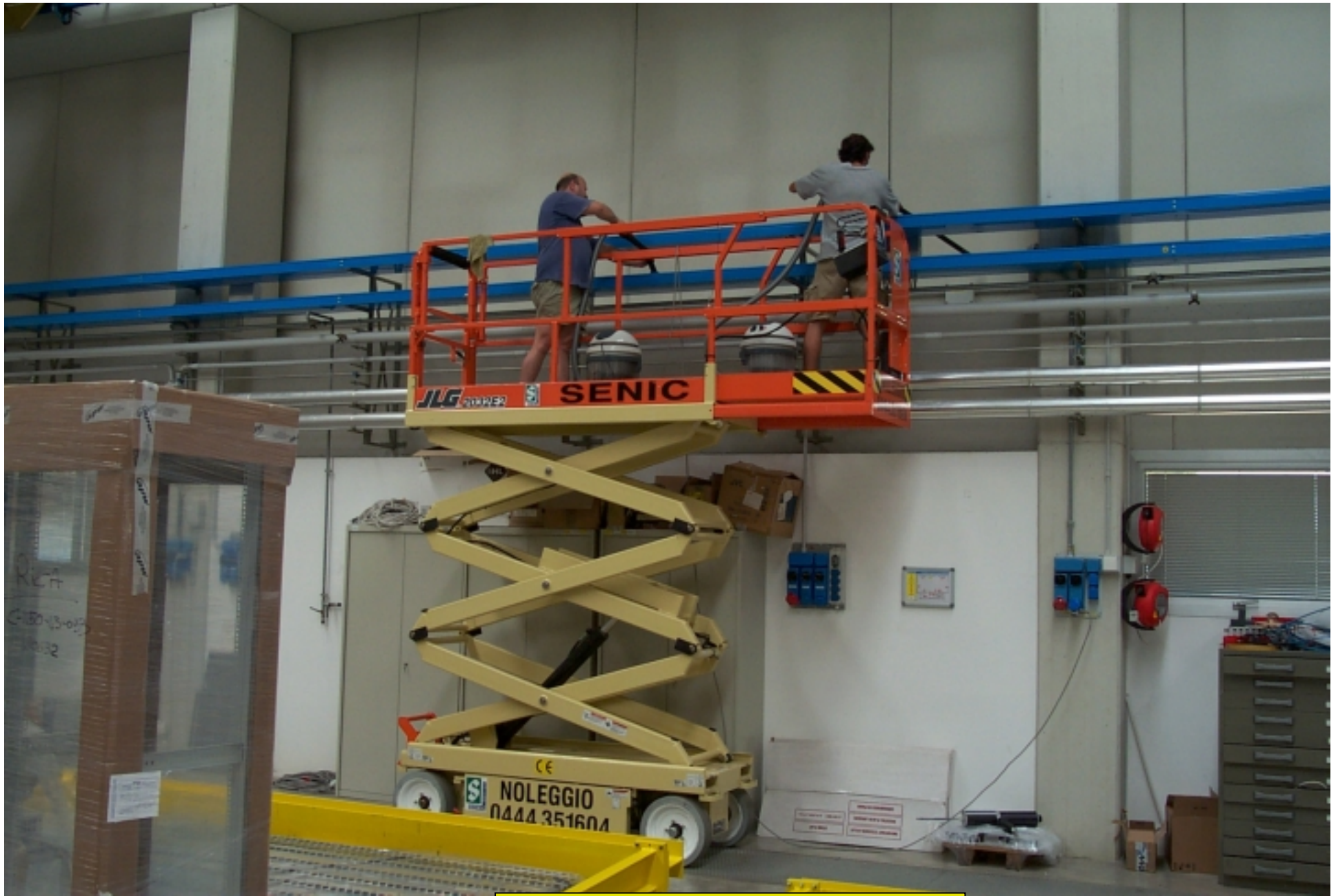
Cleaning of Legnaro hall
